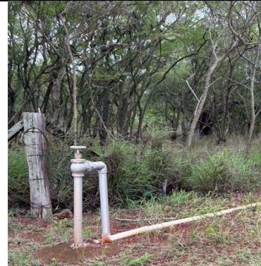
Too much volcanic rock to bury supply pipelines-
